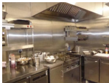
Stainless Steel Wall Cladding
